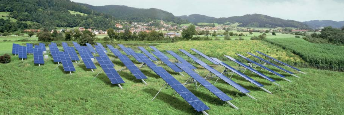
Rheinau location. 28 easily installed compact, tracking SunCarrier 22 units generate 135,000 kWh per year.
